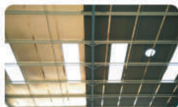
Under Roof Insulation
